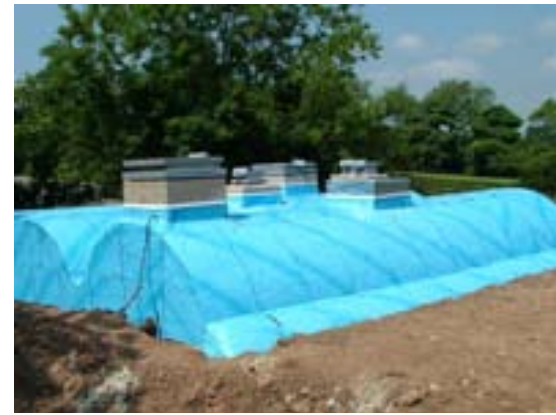
Mayfield service reservoir roof
