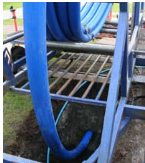
Mains replacement - pipe bursting process, minimal disruption to customers.
