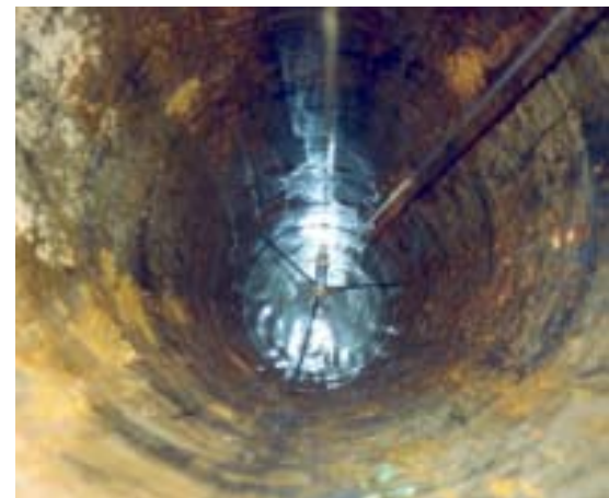
CCTV investigation used as part of the borehole maintenance process
