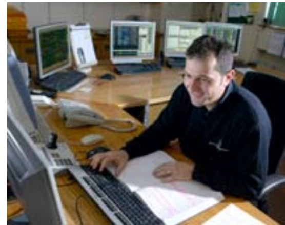
Control room at Seedy Mill Water Treatment Works
