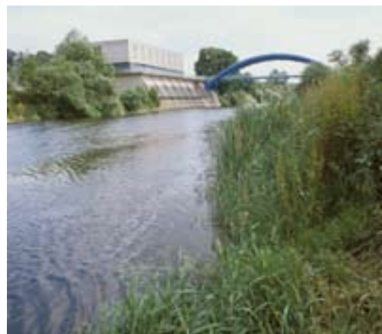
Abstraction works at the River Severn at our largest source, Hampton Loade.
